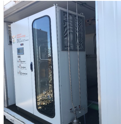
5 kW Hydrogen Fuel Cell System
