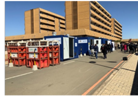
Fuel Cell deployment to power COVID-19 facilities at 1 Military Hospital, Pretoria
