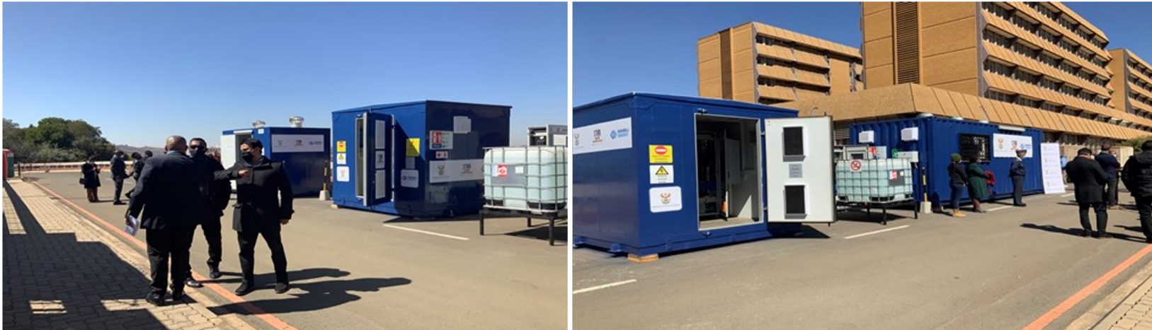
Methanol Based fuel cell systems deployed at 1 Military Hospital in Pretoria. A 5kW System will be deployed at the Ilembe District Disaster Management Centre in KwaDukuza.
