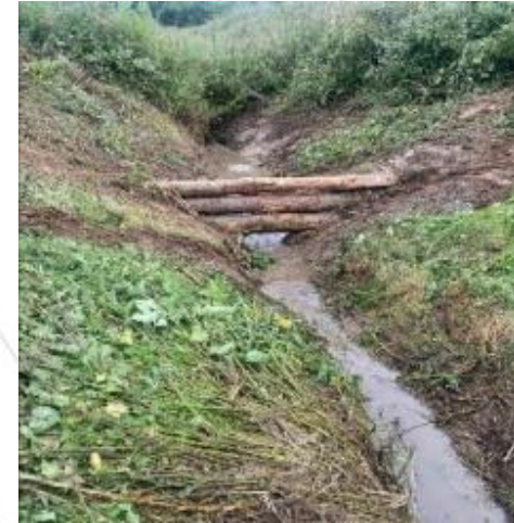
Leaky barrier in the River Lymn NFM project ©South & East Lincs Climate Action Network
