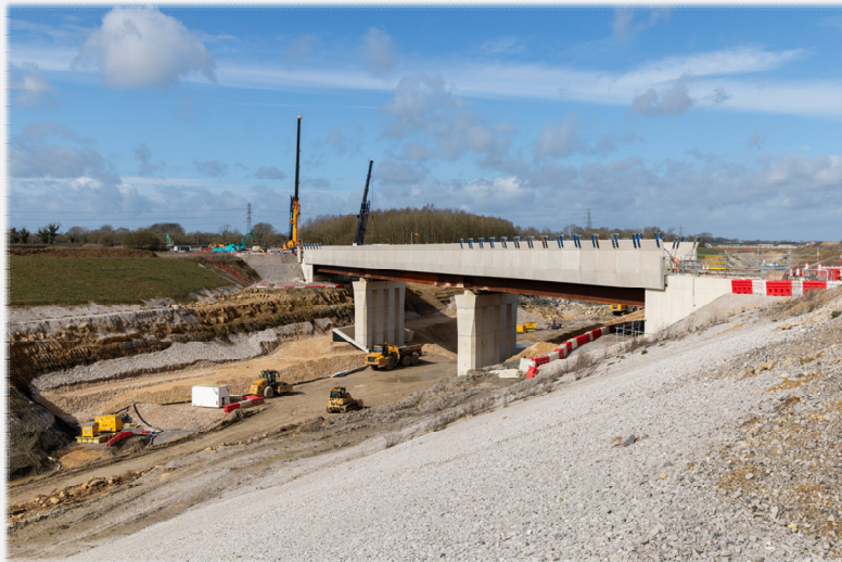
Main Work Civils
